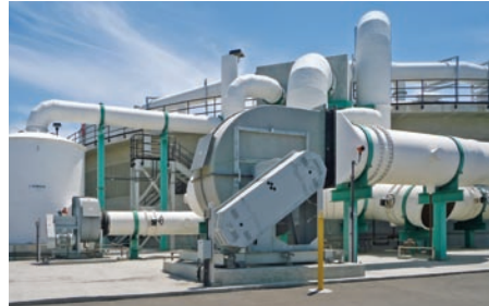
Screen washing Series 41 with odor control scrubber
